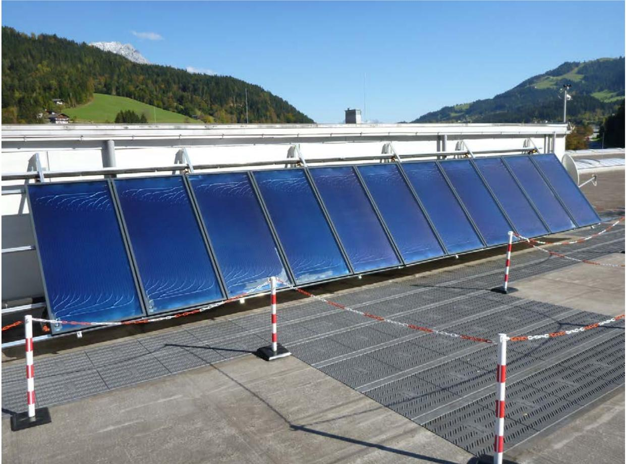
**Figure 4: The first installed and running BIONICOL field test system on the TiSUN flat roof**
